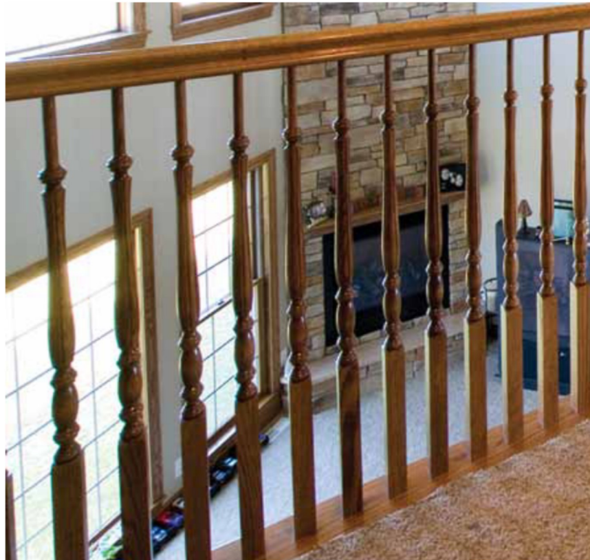
Pictured Far Right: LJ-6519P Handrail, LJF-3240 Series Newels and LJP-2105 Balusters.
